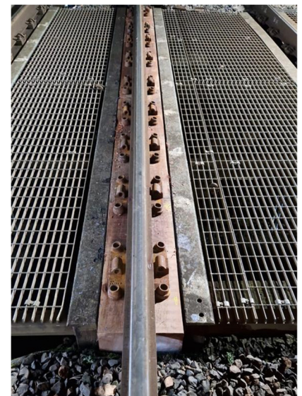
Lairds :- 4/8no. Timbers replaced
