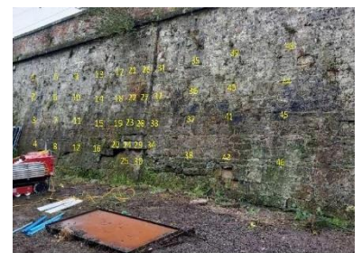
- wall monitoring points locations
